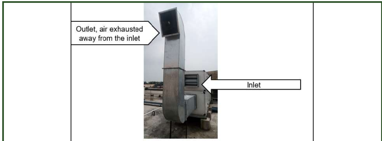
Figure 6.19: Appropriate installation of air exhaust and air inlet, HMS, Jolly Grant
